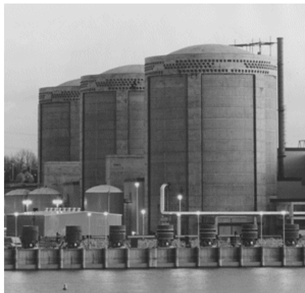
Fig. 3 Oconee Nuclear Power Station (Greenville, South Carolina) containment structures.
