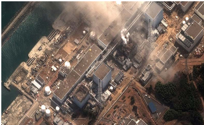
Fig. 3 Aerial image of the stricken Fukushima Daiichi nuclear power plant, showing damaged reactor buildings. (Credit: Department of Energy Aerial Measuring System)
