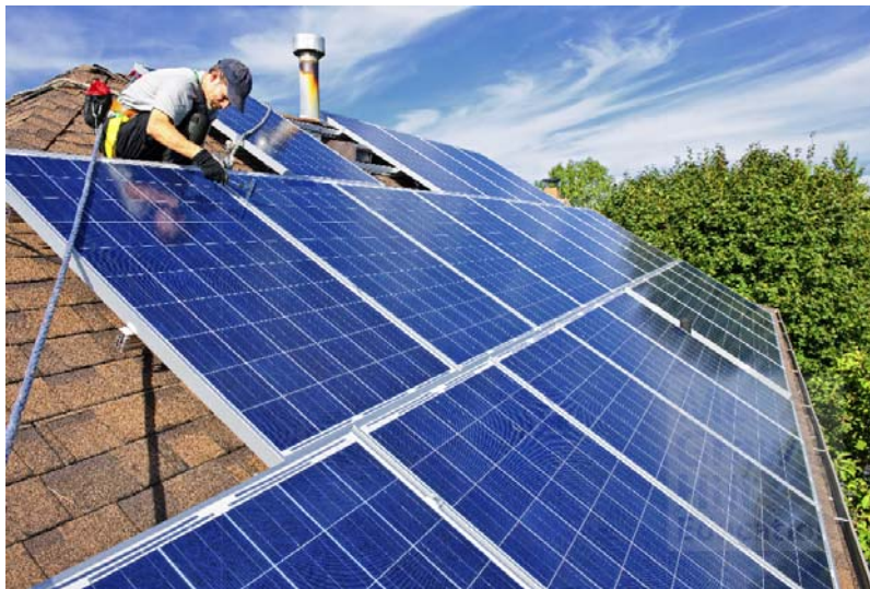
Fig. 3 Rooftop solar panel installation. (Credit: Elenathewise/Getty Images)
