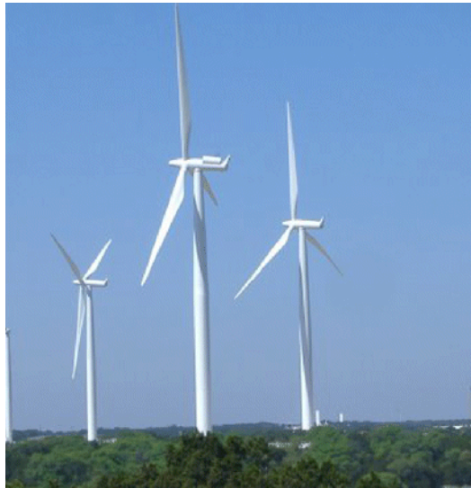
Fig. 2 Typical horizontal-axis high-power wind turbines. Such turbines can produce several megawatts of electric power depending on their size. (Credit: Department of Energy)
