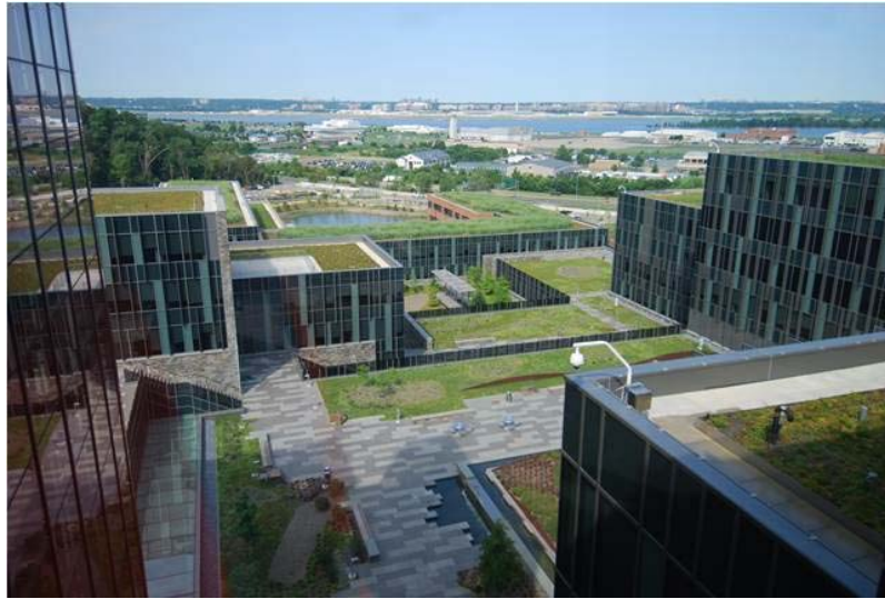
Fig. 1 Green roofs, also known as vegetated roofs or living roofs, at the U.S. Coast Guard Headquarters, Washington, DC. Engineered green roofs reduce stormwater runoff, reduce energy use through cooling effects, and provide urban habitats for plants, insects, and birds. Green roofs are also aesthetically pleasing and are expected to last about twice as long as conventional roofs. (Credit: U.S. General Services Administration)
