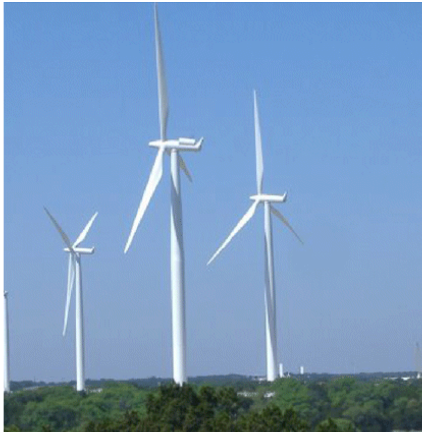
Fig. 2 Typical horizontal-axis high-power wind turbines. Such turbines can produce several megawatts of electric power depending on their size. (Courtesy of the Department of Energy)
